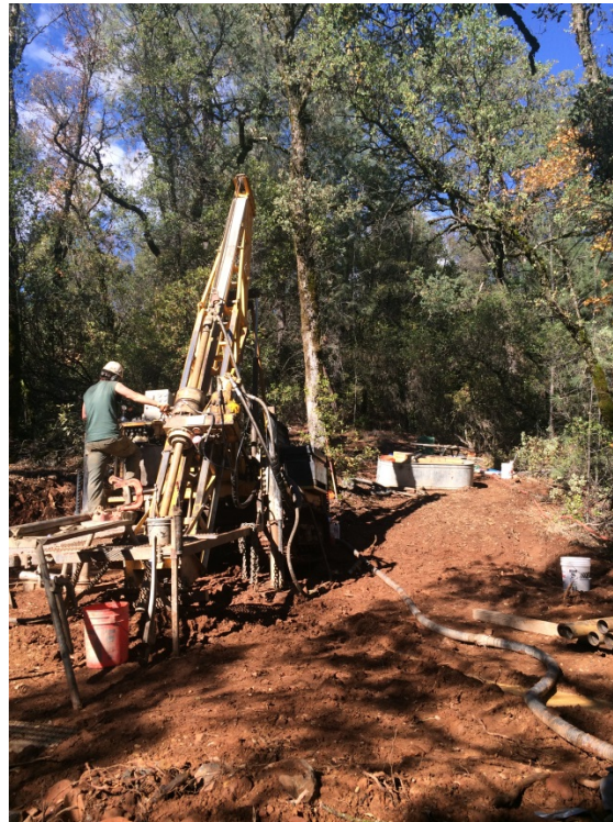
Photograph 10. Drilling Boring CB-3 (Axis 2, right abutment)
