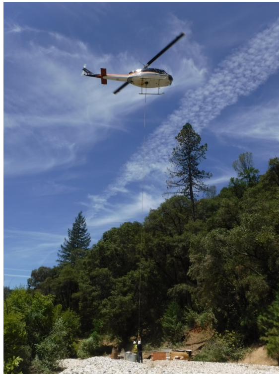
Photograph 12. Helicopter mobilization of equipment to CB-15 drill site
