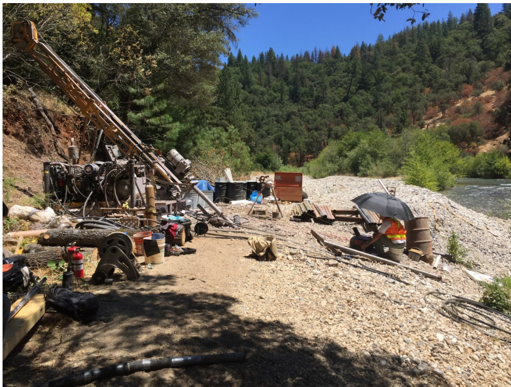
Photograph 11. Drill rig with televiewer logging at Boring CB-15
