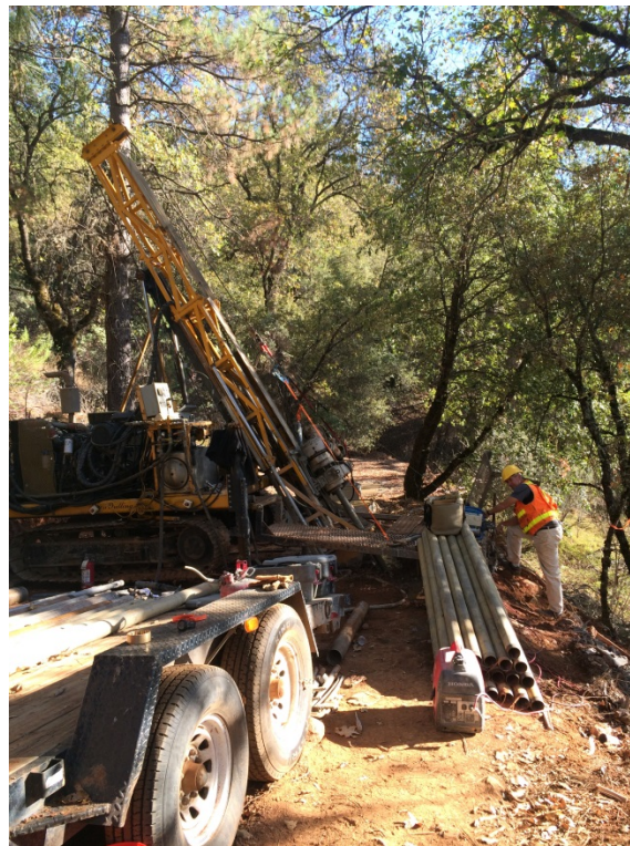
Photograph 11. Drill rig with televiewer logging at Boring CB-6 (Axis 6, left abutment)
